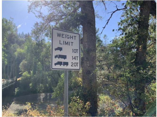
Photo 2 Load posting sign at the Abutment 2 approach
