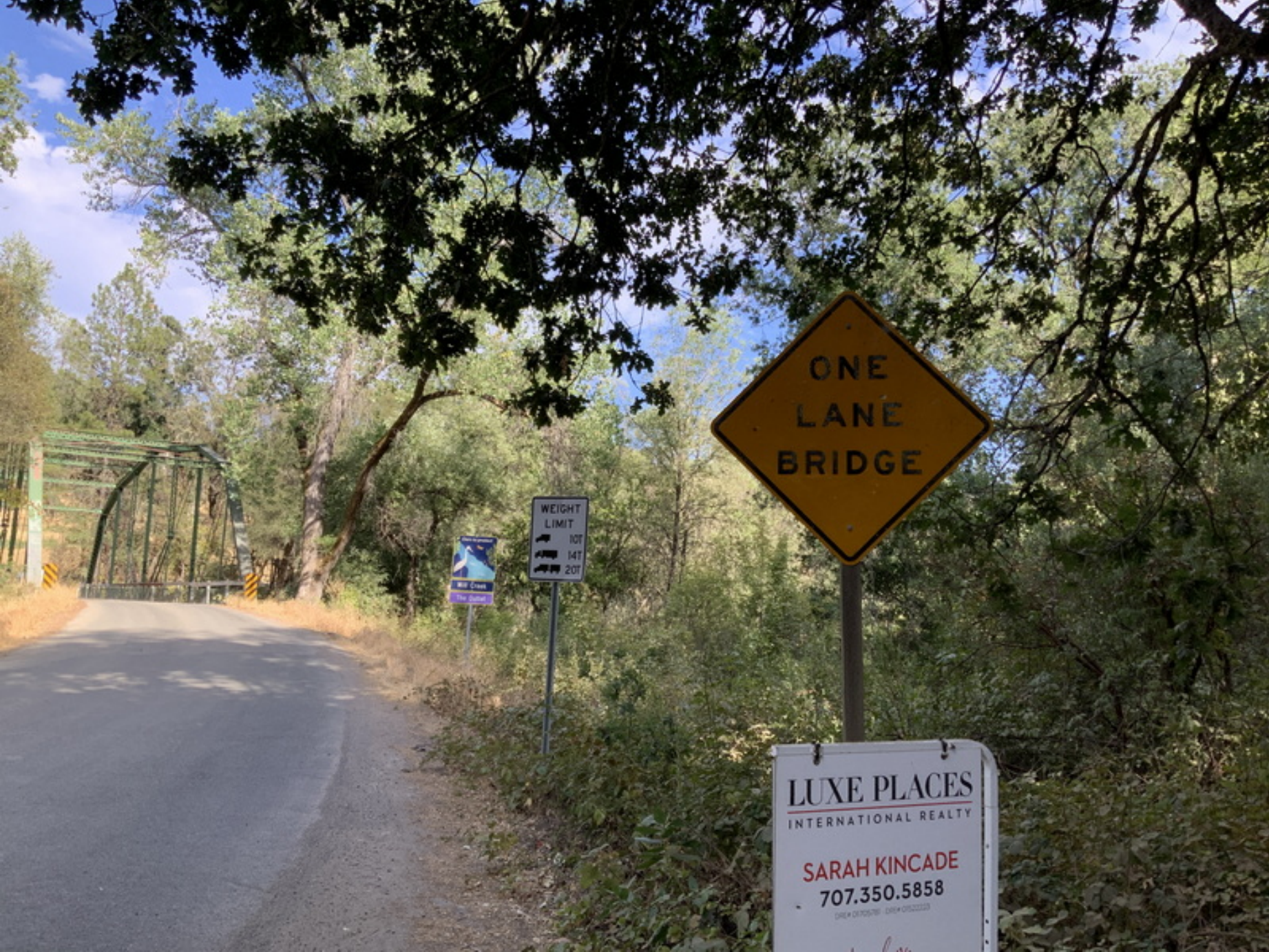
Photo #1 Operational signs at the Abutment 1 approach
