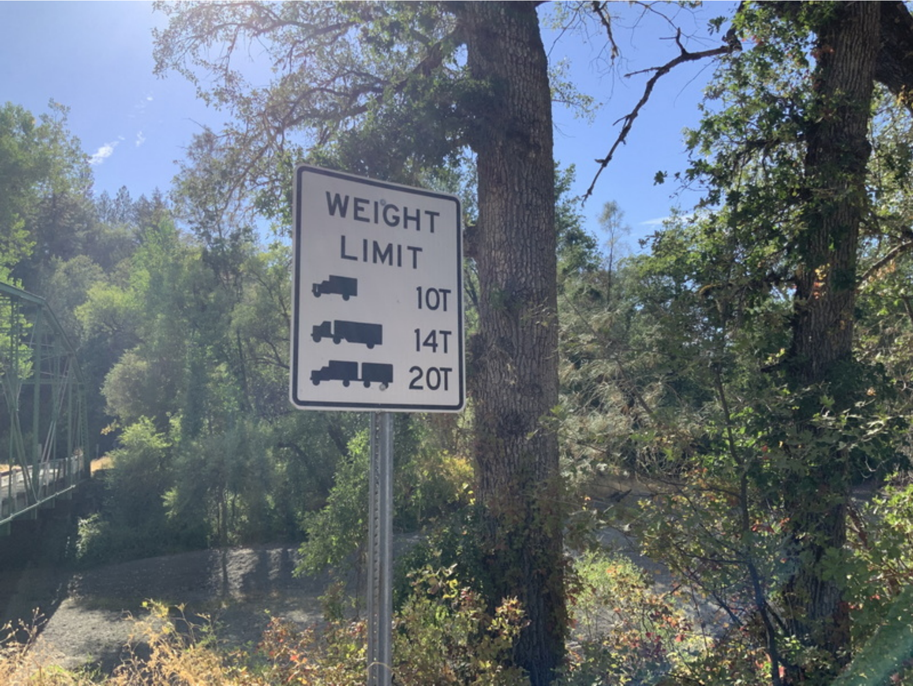
Photo #2 Load posting sign at the Abutment 2 approach
